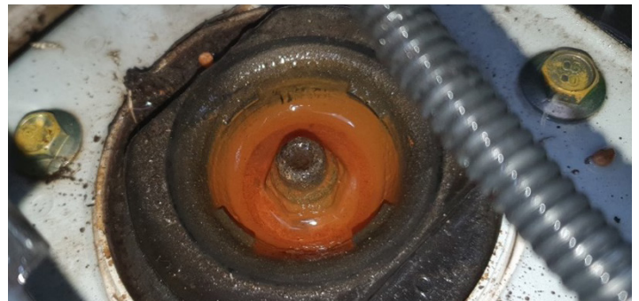
If you see any movement or corrosion in the strut assembly, check the vehicle meets the VIRM requirements before issuing a WoF.
