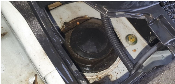
But, when the cap is removed, the corrosion damage from water shows in the upper strut mounting.
